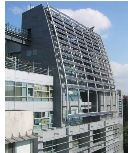
Fu-Bon Memorial Building: 19.8 kW
