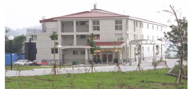
RDF demon plant in Hualien BOE Project, Tech. developed by ITRI
