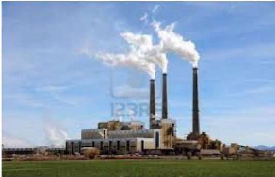
Flexible Dispatchable Generation (Natural Gas and (gasp!) Diesel Plants)
