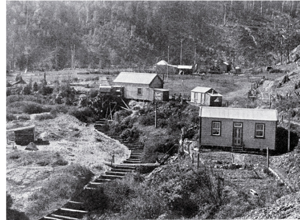
The electric light power house, Reefton
