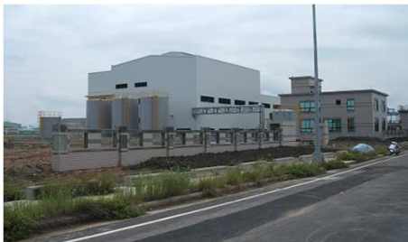
Commercial bio-diesel plant (10,000 kL/yr in Changhua , 2007)
