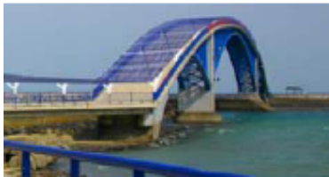
Bridge with Photovoltaics
