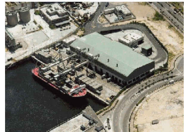
The West Kowloon Transfer Station
