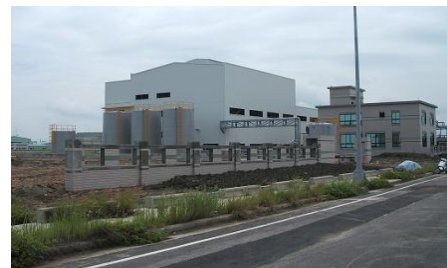
Commercial bio-diesel plant (10,000 kL/yr in Changhua, 2007)
