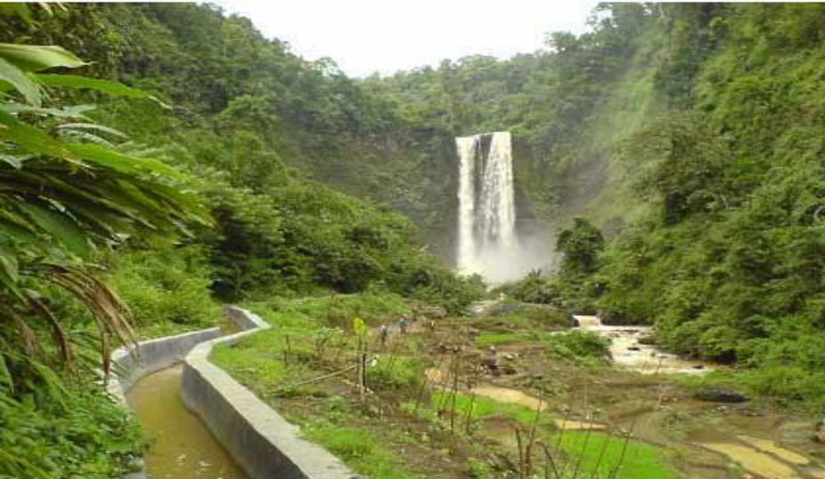
Run-off-river MHPP at water fall creek, Garut, West Java, cap. of 165 kW
