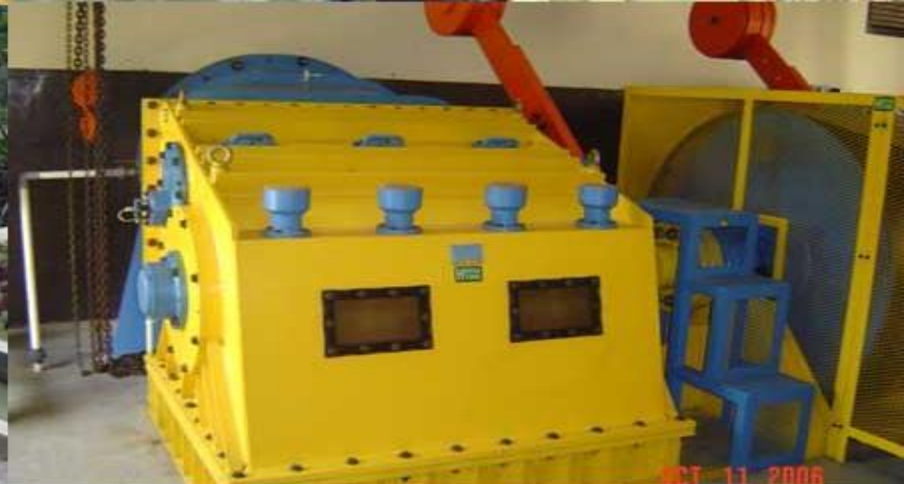
Run-off-river MHPP at irrigation system, Subang, West Java, cap. of 100 kW
