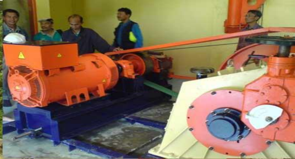
Run-off-river MHPP at water fall creek, Garut, West Java, cap. of 165 kW
