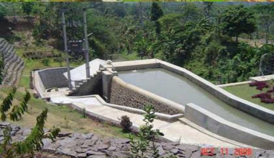
Run-off-river MHPP at irrigation system, Subang, West Java, cap. of 100 kW
