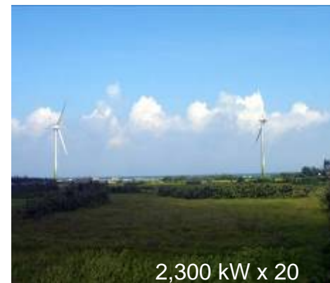
Taichung City Wind Farm Infra Vest Co. (VWing AG) (46 MW, 2008)
