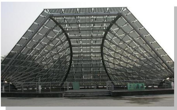
BIPV demonstration system
