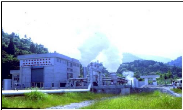
Chingshui Geothermal Power Plant
