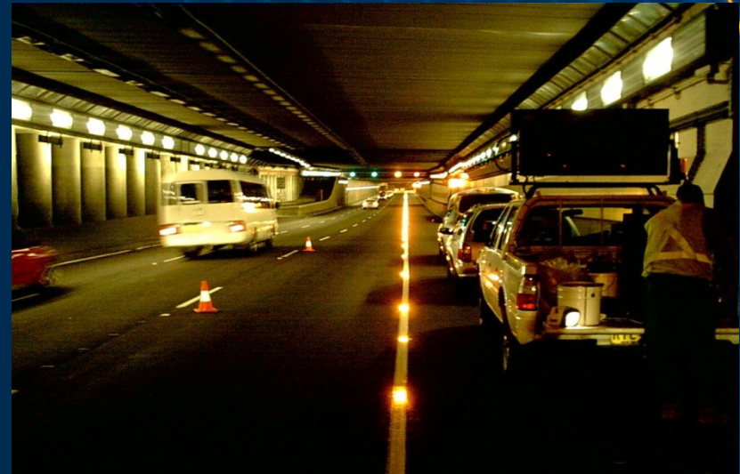
Tunnel (Sydney Australia)
