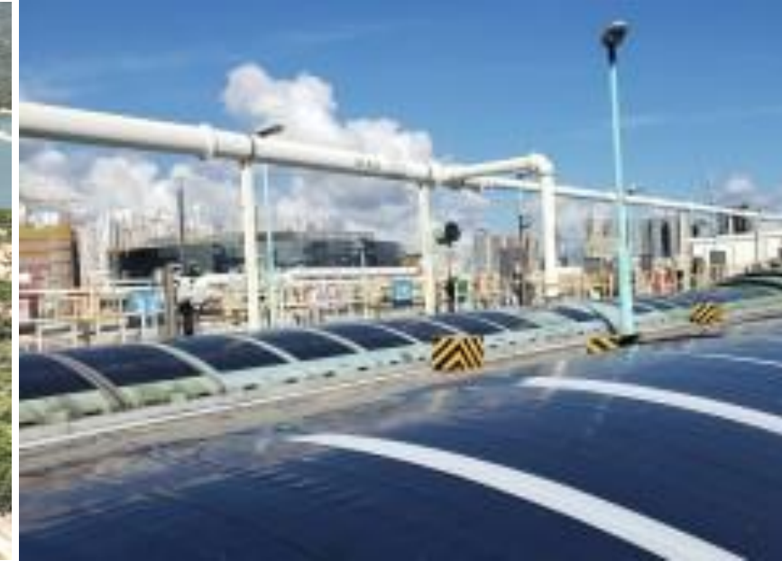
Thin-film system at Stonecutters Island Sewage Treatment Works
