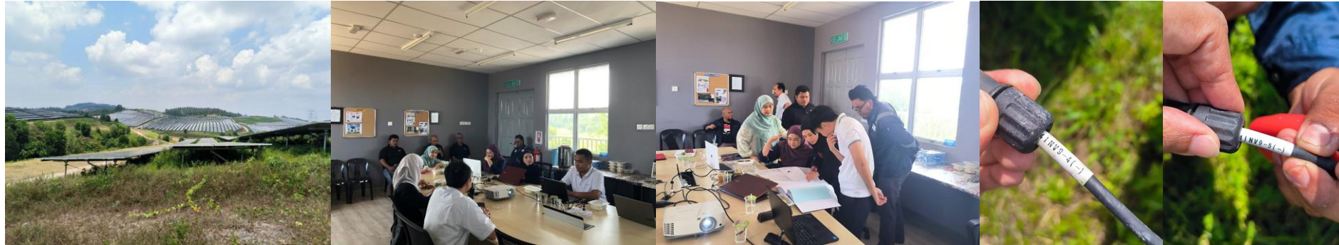
25MW AC large-scale solar photovoltaic power plant in Pasir Gudang, Malaysia
