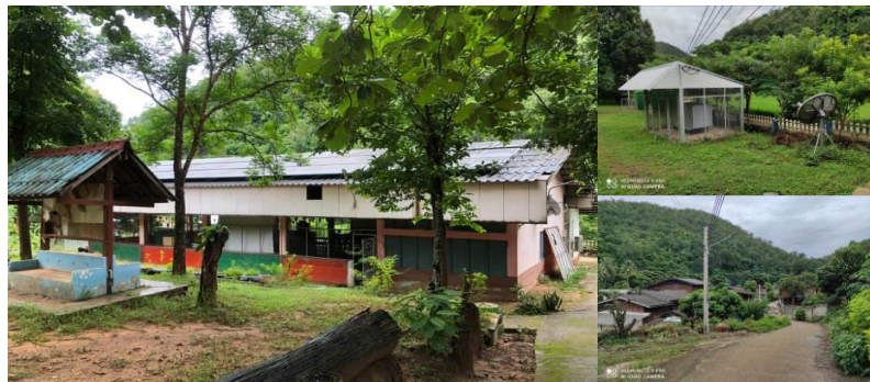
100-kW microgrid at Ban Pha Dan, Lamphun | rural microgrid
