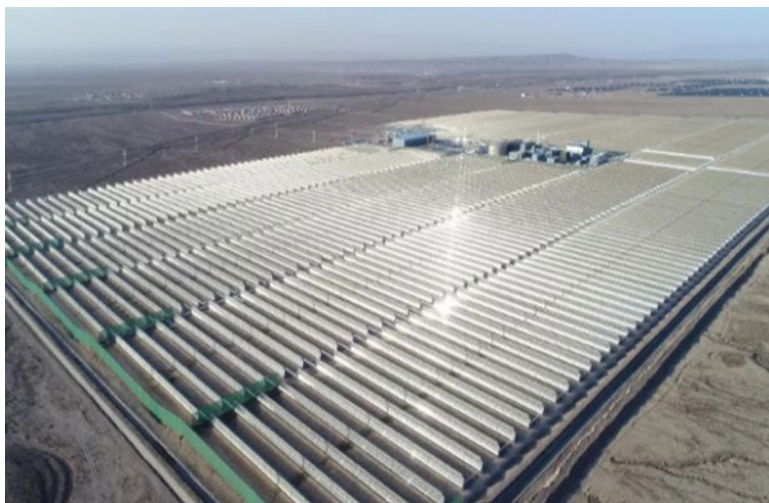
中广核德令哈50MW槽式光热电站 Delingha 50MW parabolic trough power plant
