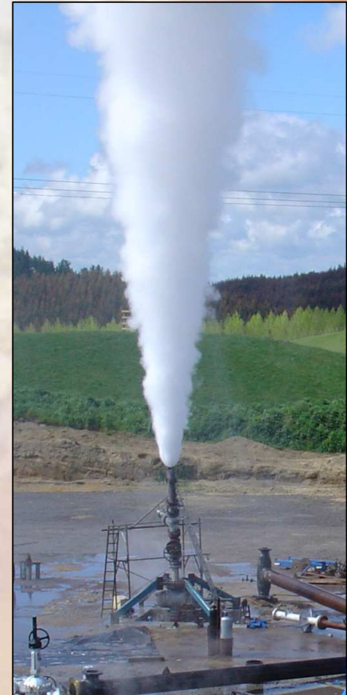
Drilling ignimbrite-hosted high temperature geothermal systems of the TVZ
