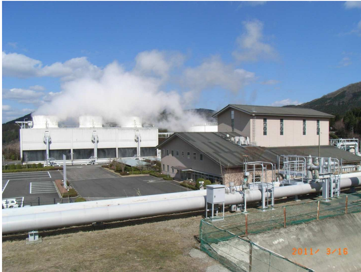
Takigami Power Station of Kyushu Electric Power Co., Inc. and Idemitsu Oita Geothermal Co., Ltd
