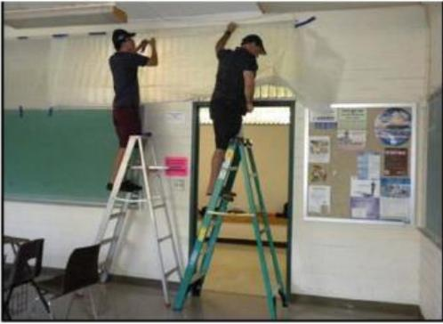
Installing the temporary tarp to seal sections of the louvered openings; seen from classroom 302
