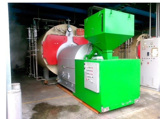
Bio-pellet-fired boiler
