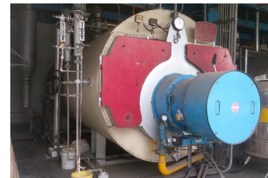
Natural-gas-fired boiler
