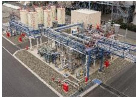
At the hydrogenation plant, hydrogen and toluene are chemically converted to MCH, which is then shipped to Japan by sea and converted back to hydrogen and toluene at the dehydrogenation plant in Kawasaki.
